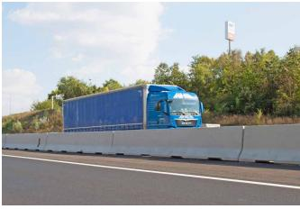
Containment level Working width Impact severity level H3 (covers H2, H1, N1, T3, T2 and T1)
