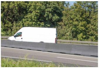
Containment level Working width Impact severity level H4b (covers H3, H2, H1, N1, T3, T2 and T1) W5 (covers W6, W7 and W8) ASI B
