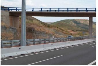
Containment level Working width Impact severity level H2 (covers H1, N1, T3, T2 and T1) W1 (covers W2, W3, W4, W5, W6, W7 and W8) ASI B
