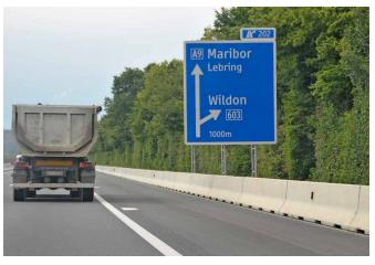
Containment level Working width Impact severity level H2 (covers H1, N1, T3, T2 and T1) W5 (covers W6, W7 and W8) ASI B
