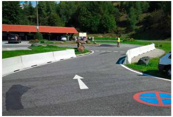
Containment level Working width Impact severity level N2 (covers N1, T2 and T1) W4 (covers W5, W6, W7 and W8) ASI B
