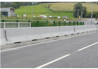
**Containment level** Working width Impact severity level **H2** (covers H1, N1, T3, T2 and T1) W2 (covers W3, W4, W5, W6, W7 and W8) ASI B
